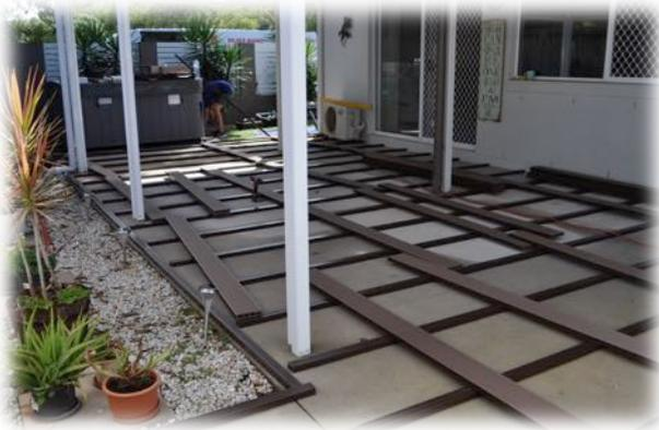
ECW Joists screwed on concrete, spaced 550mm apart
