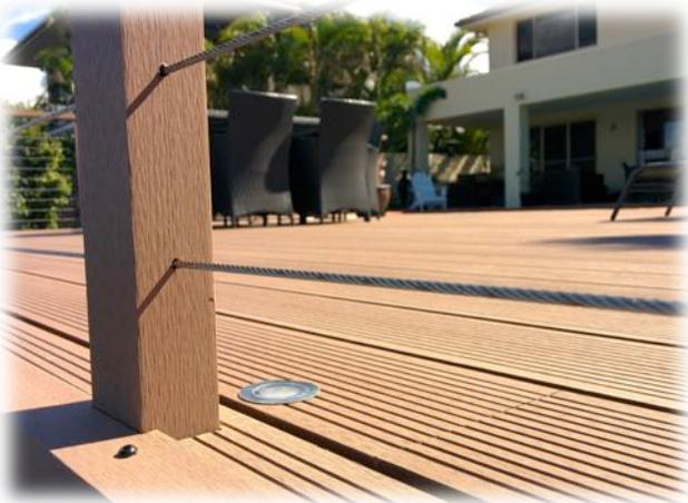
Composite balustrade and handrail with made 60x40 columns and stainless steel wire rope
