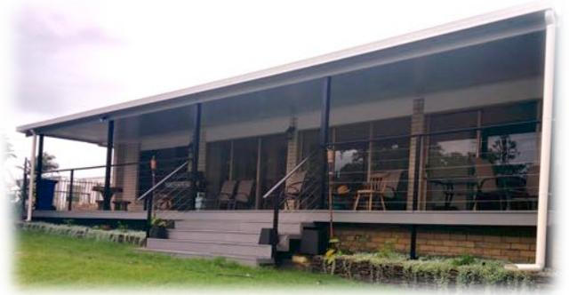
Another option is to use powder coated aluminium balustrade and handrail with stainless steel wire rope (picture above). The deck was built with Light Grey boards and black balustrade for contrast.
